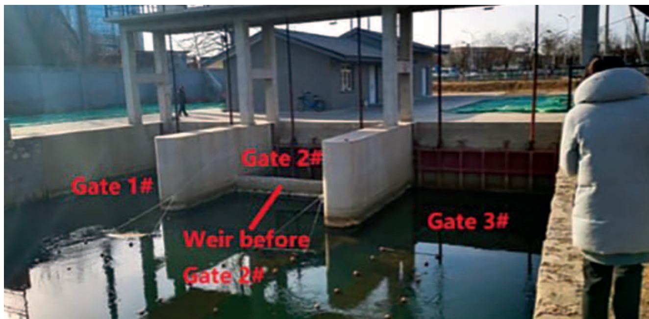
Figure 8 Overflow structure Yudai River Channel with gates (old state); overflow weir in the center 图 8 带闸门的玉带河溢流结构（水泰和设备安装前）；溢流堰位于中心
